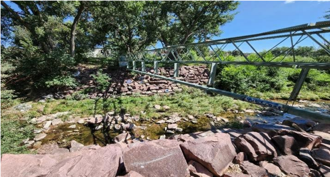
Figure 34: Photo of existing aerial sanitary sewer line.
