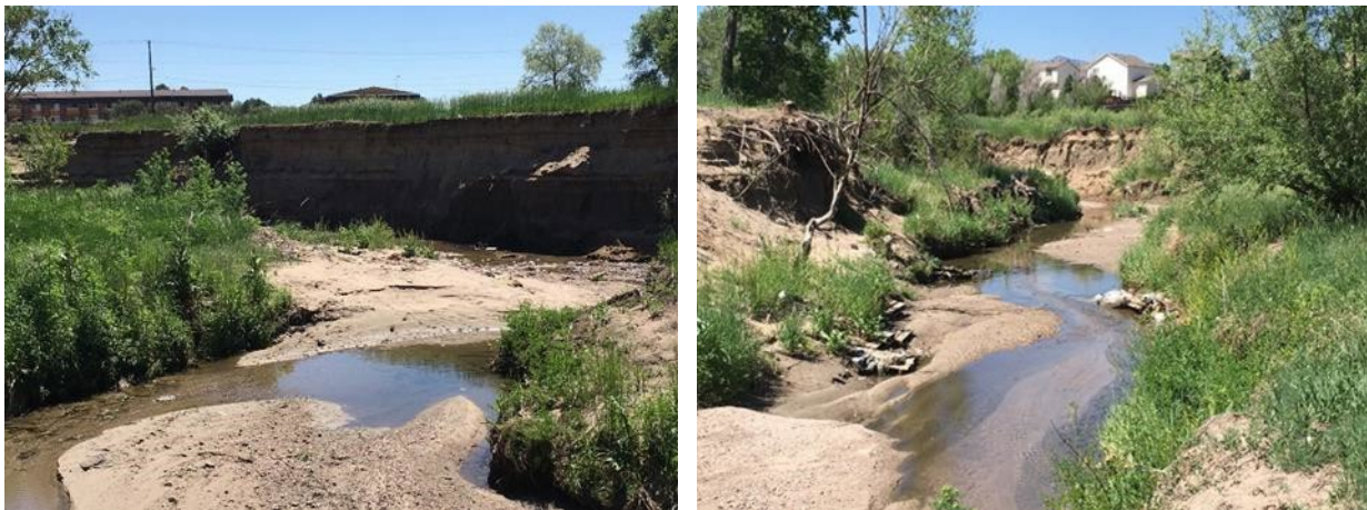
Figure 7: Photos of Reach 2 showing the stream incision. (Date: 2022)
